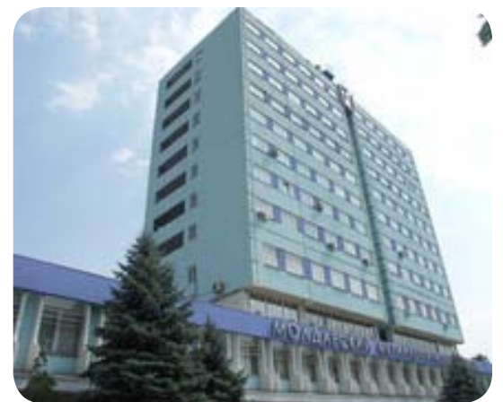
Moldova Steel Works
